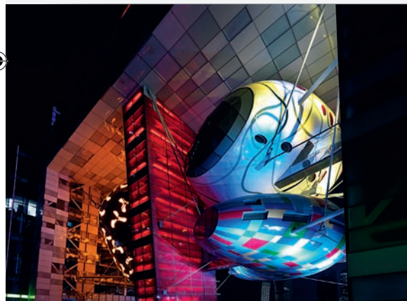
Curran says that the concept for the Shanghai Chandelier was born out of a site constraint—two vehicular tunnels pass through the middle of the site, crossing underneath the Huangpu River all the way to Pudong on the other side, making it a no-build zone. Spark decided to turn the constraint into an opportunity, creating an “arch gateway overlooking the waterfront” as the structure for the Chandelier
